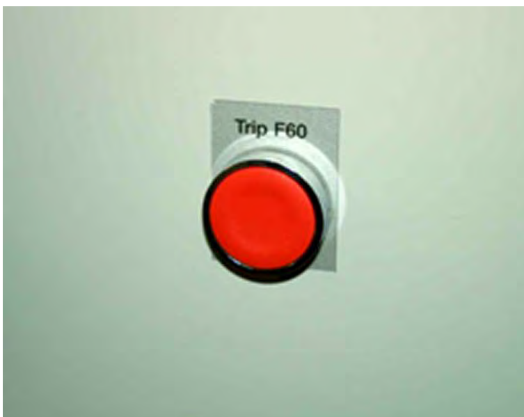
Picture 6 The trip F60 button (pos. 5, Figure 1)
